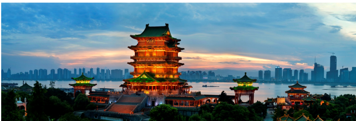
Description: Pavillon of Prince Teng, Nanchang Copyright: Nanchang DRC
